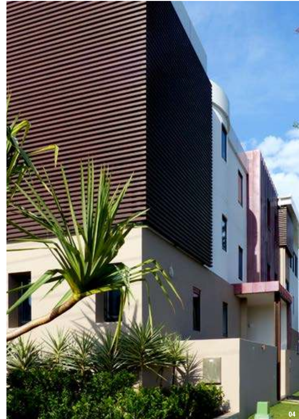
01: RHS Geometric 150mm x 50mm. Colour: Kwila 02: Battens 100mm x 50mm. Colour: Atlantic Cedar 03: Battens 50mm x 50mm. Colour: Bush Cherry 04: Battens 50mm x 50mm. Colour: Kwila
